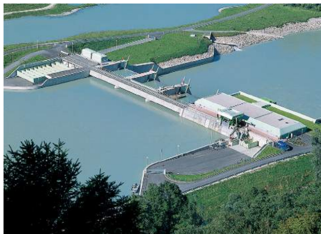
FIG. 3— Hydro power plant.
